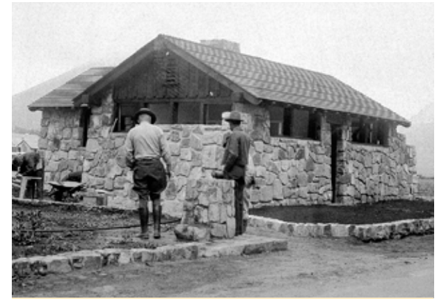
CCC-built "comfort station," ca. 1934
